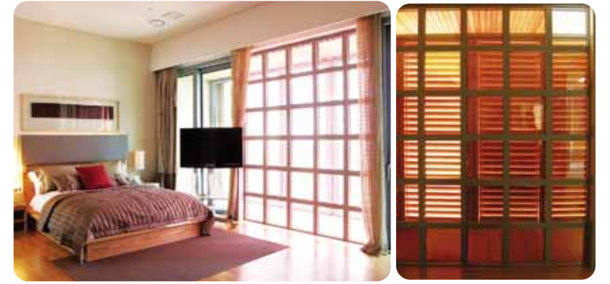
● DSSC(30 modules measuring 37x40cm 2 ) installed in the master bedroom window of the ecofriendly "Green Tomorrow" home built by Samsung Corp. Developed by Samsung SDI, the waffle-shaped windows feature the world's largest area dye-sensitized solar cells using photosensitive dyes. Transparent windows can be realized depending on the color of the dye. Unlike conventional thin film solar cells, these cells allow residents to enjoy the outside view. Moreover, electricity can be generated even on a cloudy day or with the use of artificial lighting.
